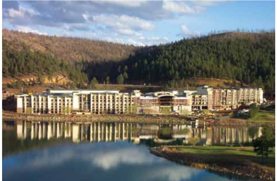
The Inn of the Mountain Gods Hotel and Casino in Mescalero, New Mexico. The $250m project had $4.5m of fireproofing work and the largest underground steel parking structure ever built in the United States.
