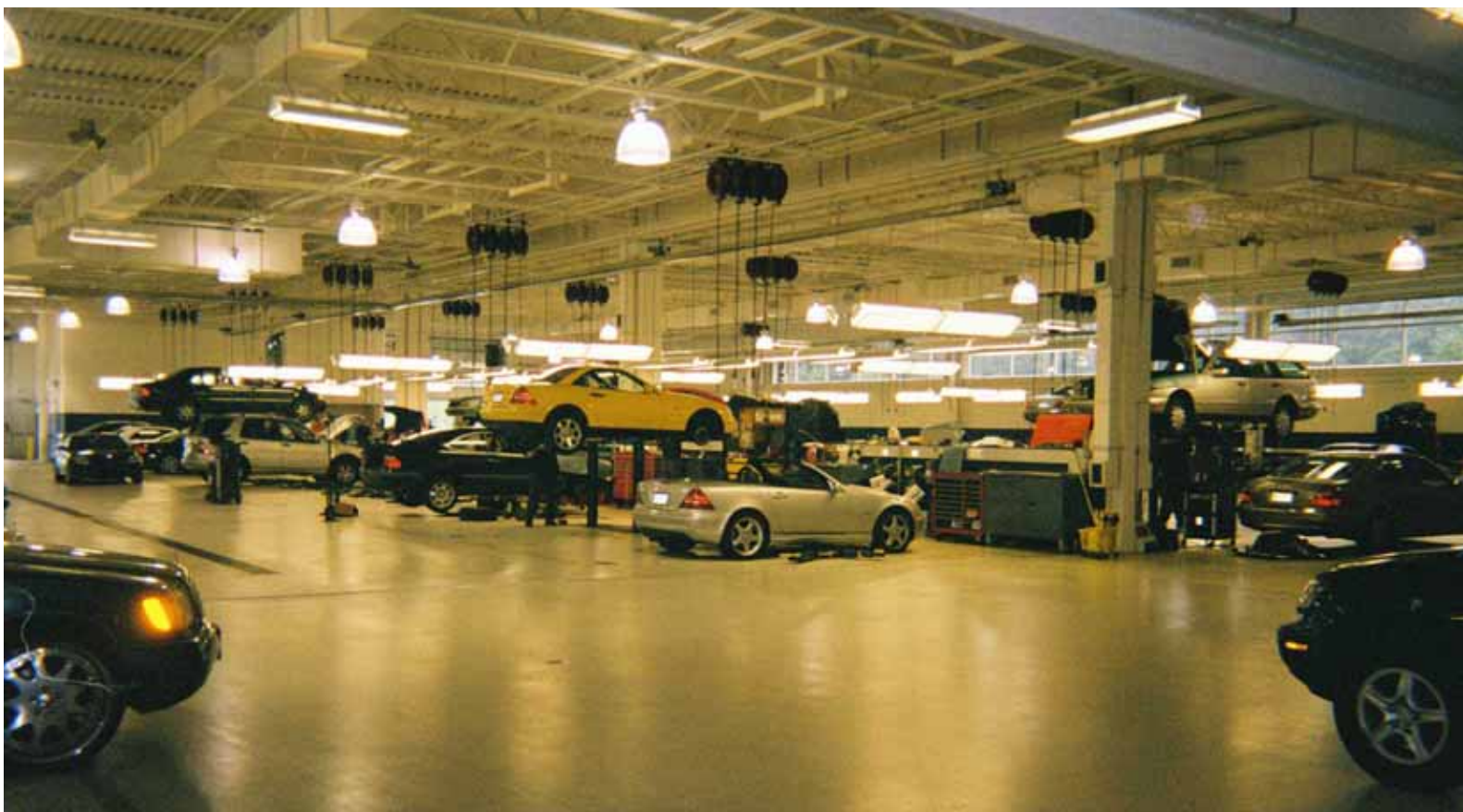
Reduced column footprints achieved with Nullifire S606 allowed for more space in the vehicle service bays. Vehicle exhaust soot can be easily wiped off the intumescent finish.
