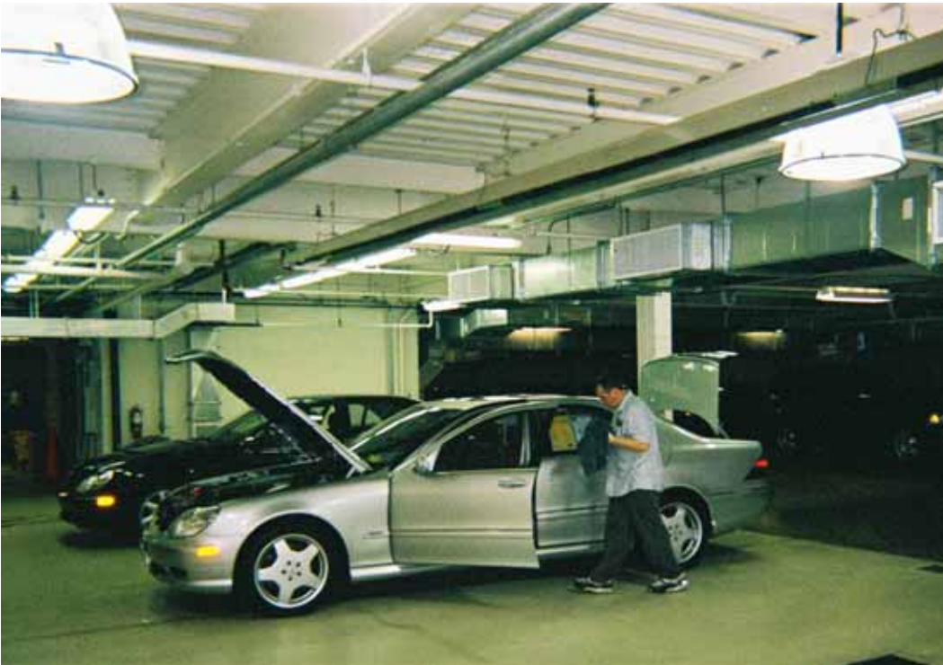
Mercedes Benz needs to store their high value inventory indoors in a basement level parking area. The floor area saved on the column footprints by going with a thin-film intumescent fireproofing product allowed for several extra parking spaces.
